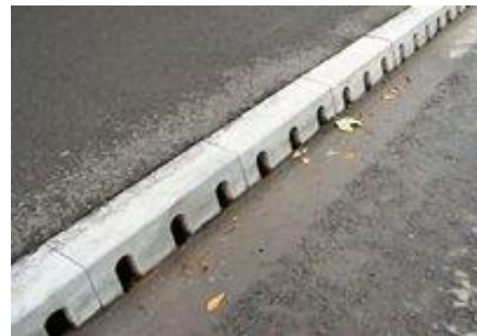
Typical Kerb Drains
