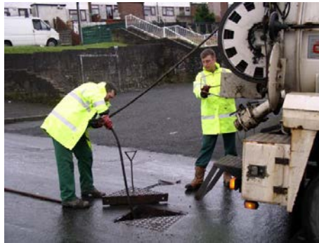
A Gully-emptier Lorry in action – cleaning a gully and jetting a manhole
